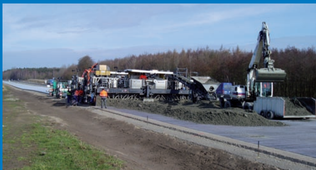
The SP 1500 L is a complete paving train, making it an ideal candidate for paving motorway carriageways. It comprises two two-tracked machines, and is fully equipped for dual-layer paving of motorway carriageways.
